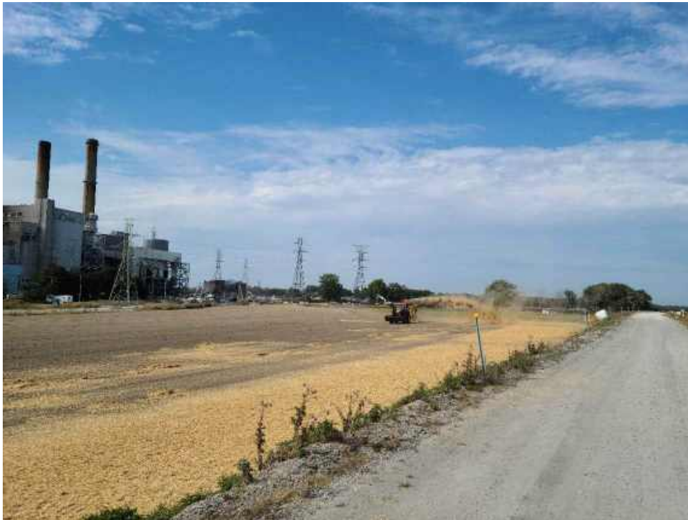
Photo 1: Fisher placing straw mulch in the north end of the restoration.
