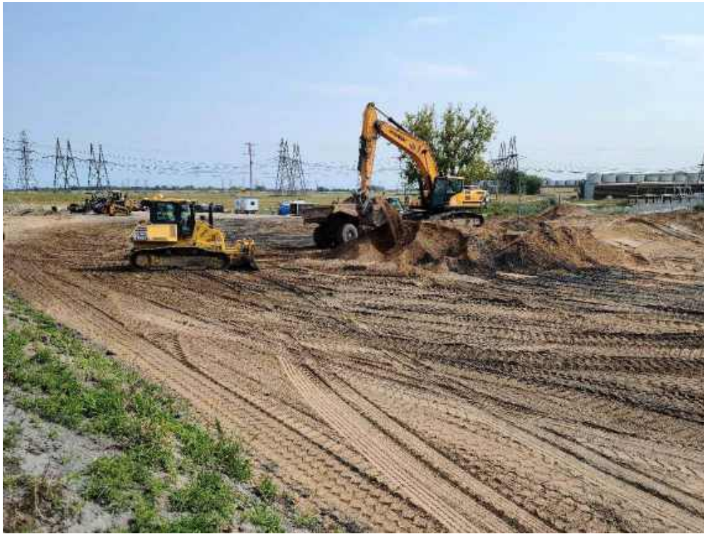
Photo 1: Fisher loading out excess berm materials.
