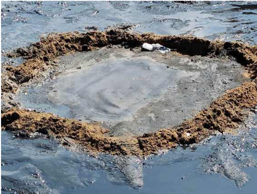
Photo 1: The repair of the perforations through the primary geomembrane.
