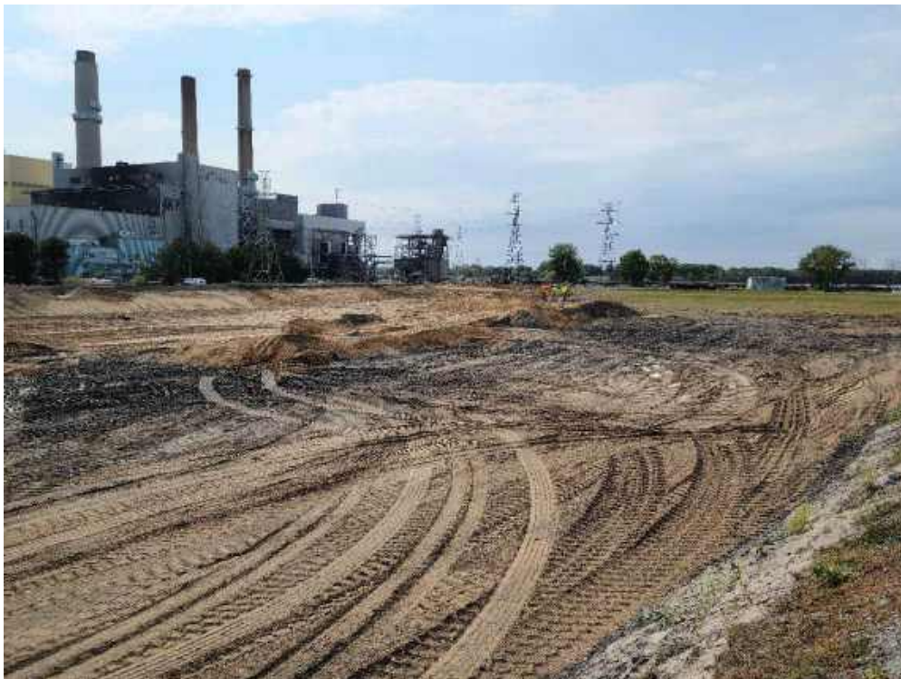
Photo 2: The primary and secondary liner systems have been removed from the Settling Basin.
