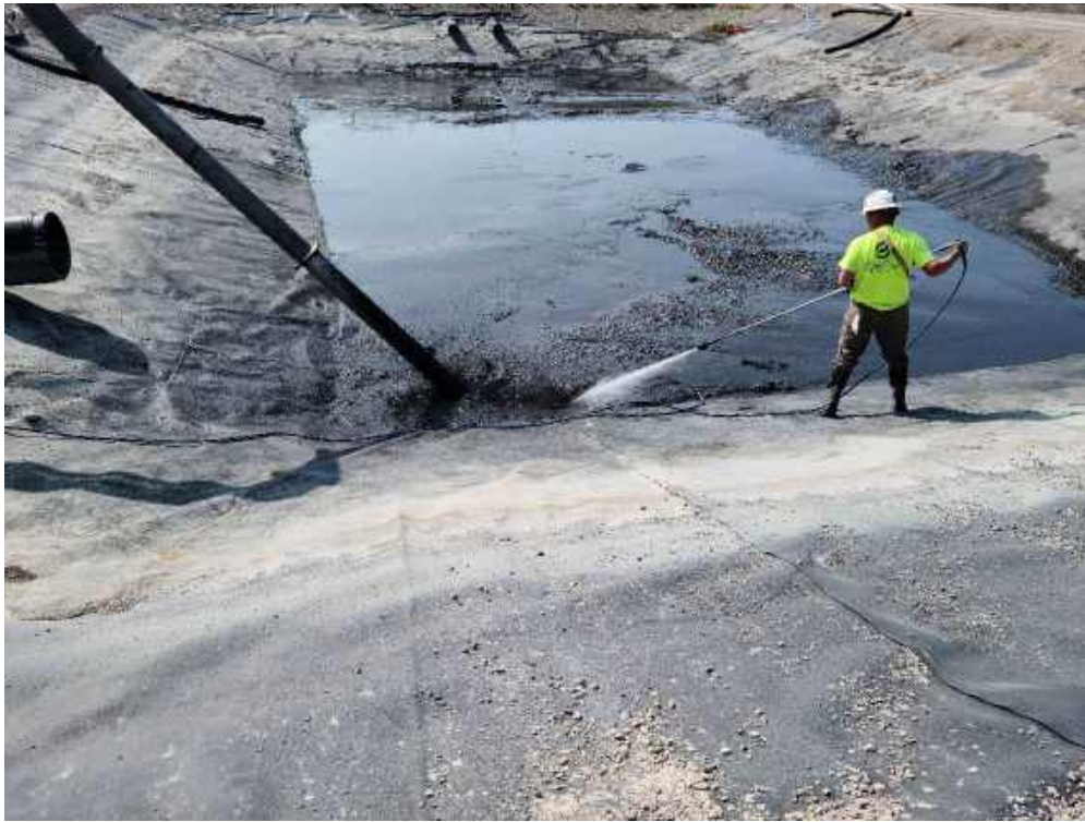
Photo 1: Badger cleaning the ash and water from the Polishing Basin.
