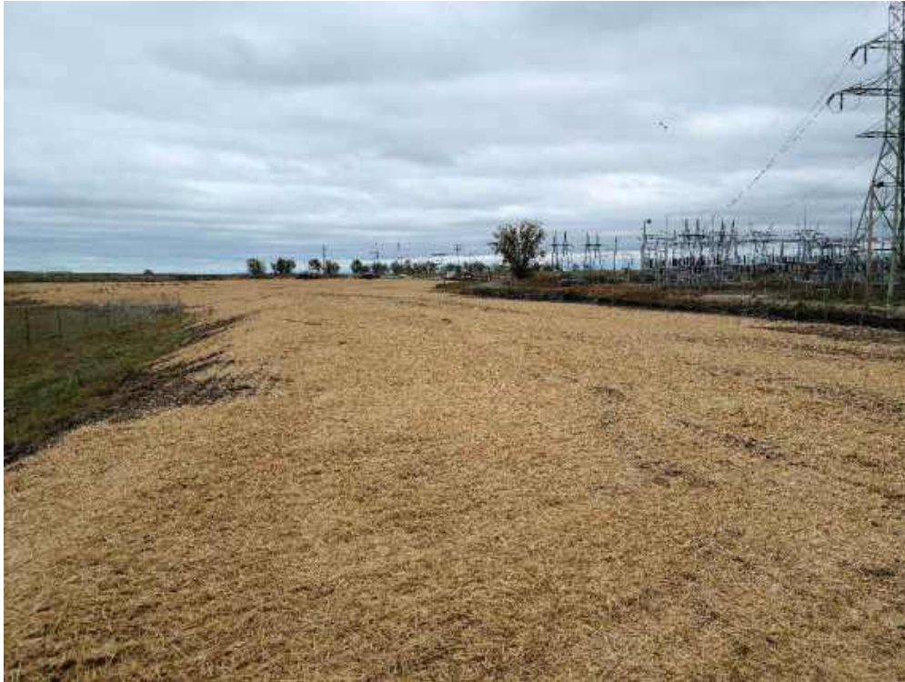
Photo 1: Photo of the restoration from the west end looking east.
