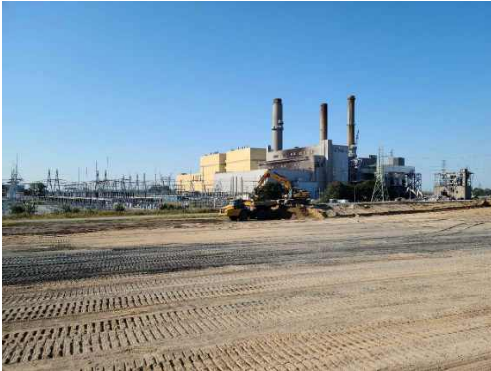
Photo 1: Fisher excavating excess berm material for disposal at the JCW Landfill.
