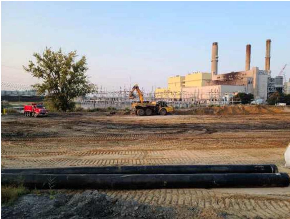
Photo 1: Fisher excavating the excess berm materials for disposal at the JCW Landfill.
