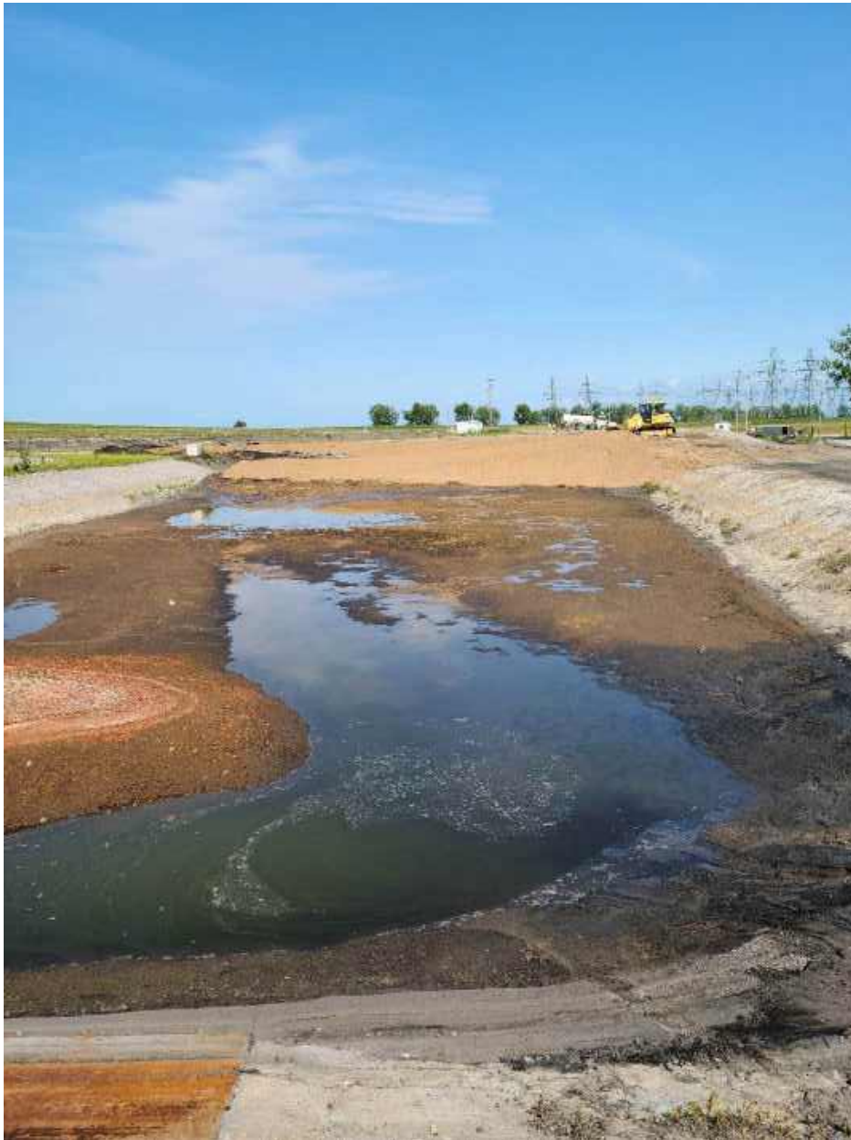
Photo 1: Fisher installing sand fingers into the Settling Basin for access.
