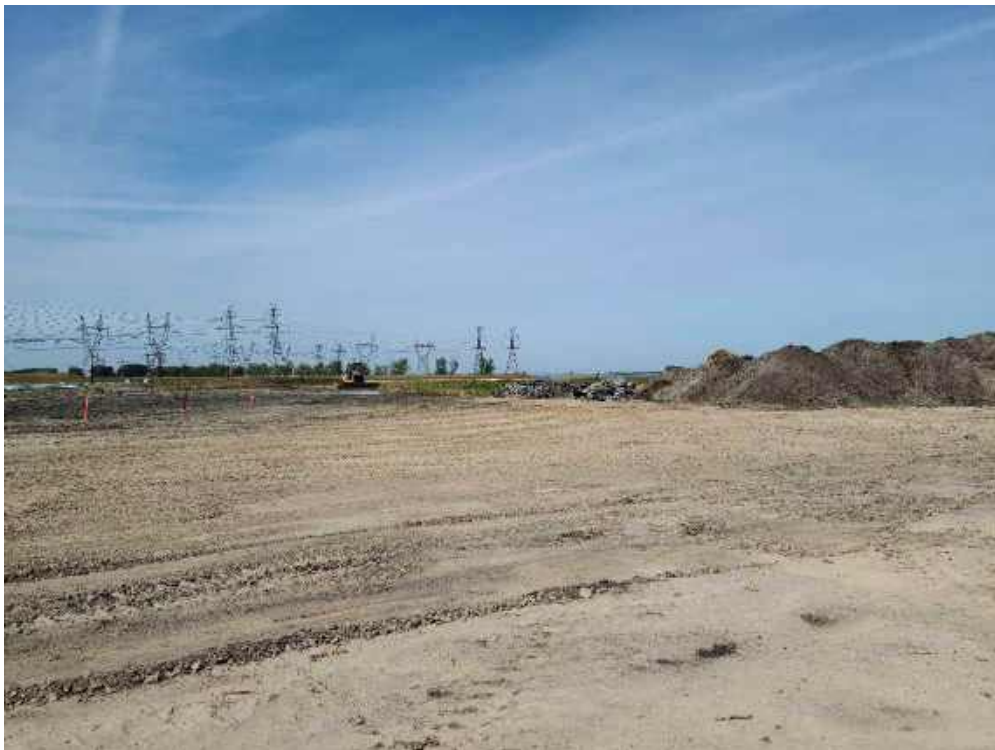
Photo 2: Fisher grading the concrete and liner/GCL fill in the JCW Landfill.
