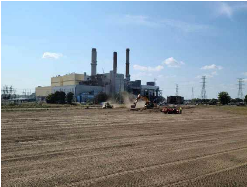
Photo 1: Fisher finishing the topsoil placement on the west end of the restoration.
