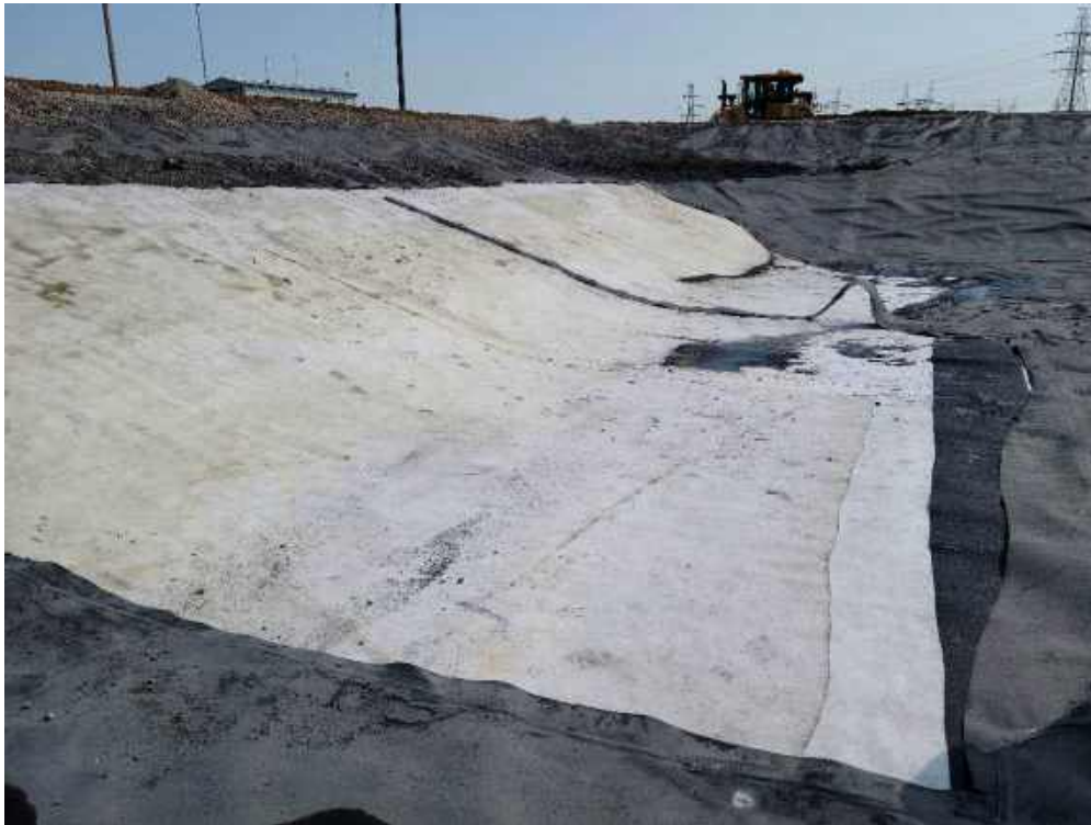
Photo 1: Fisher started removing the geomembrane liner from the Polishing Basin.
