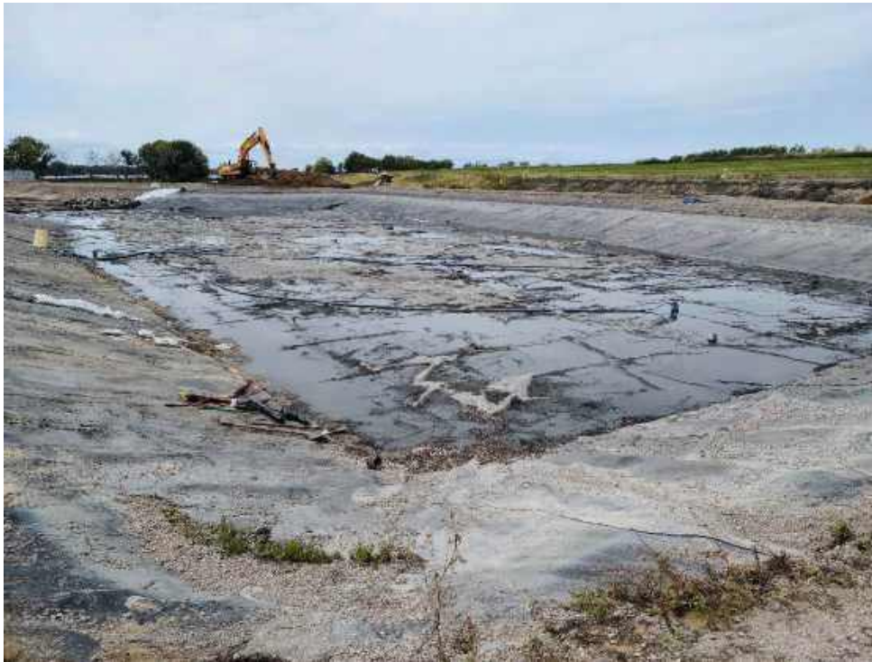
Photo 1: The Settling Basin was cleaned of ash and dewatered.
