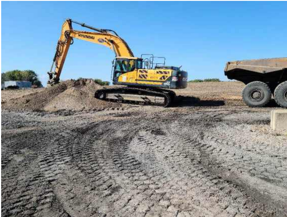
Photo 1: Fisher loading out the last of the berm material.
