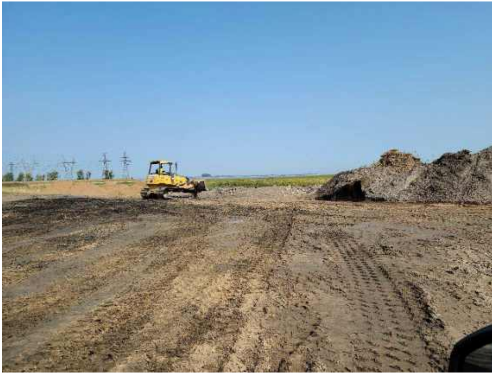
Photo 1: Fisher covering the concrete, liner, and GCL in the JCW Landfill.
