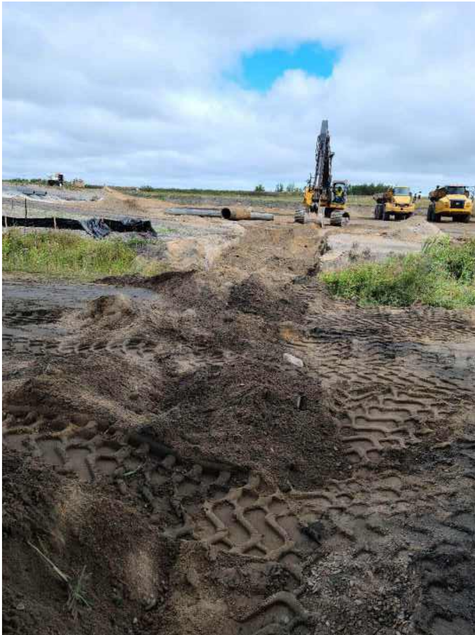
Photo 2: Fisher removed the discharge piping from the Polishing Basin.
