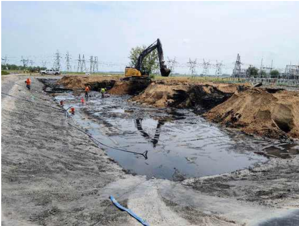
Photo 1: Fisher's progress on ash removal from the Settling Basin.
