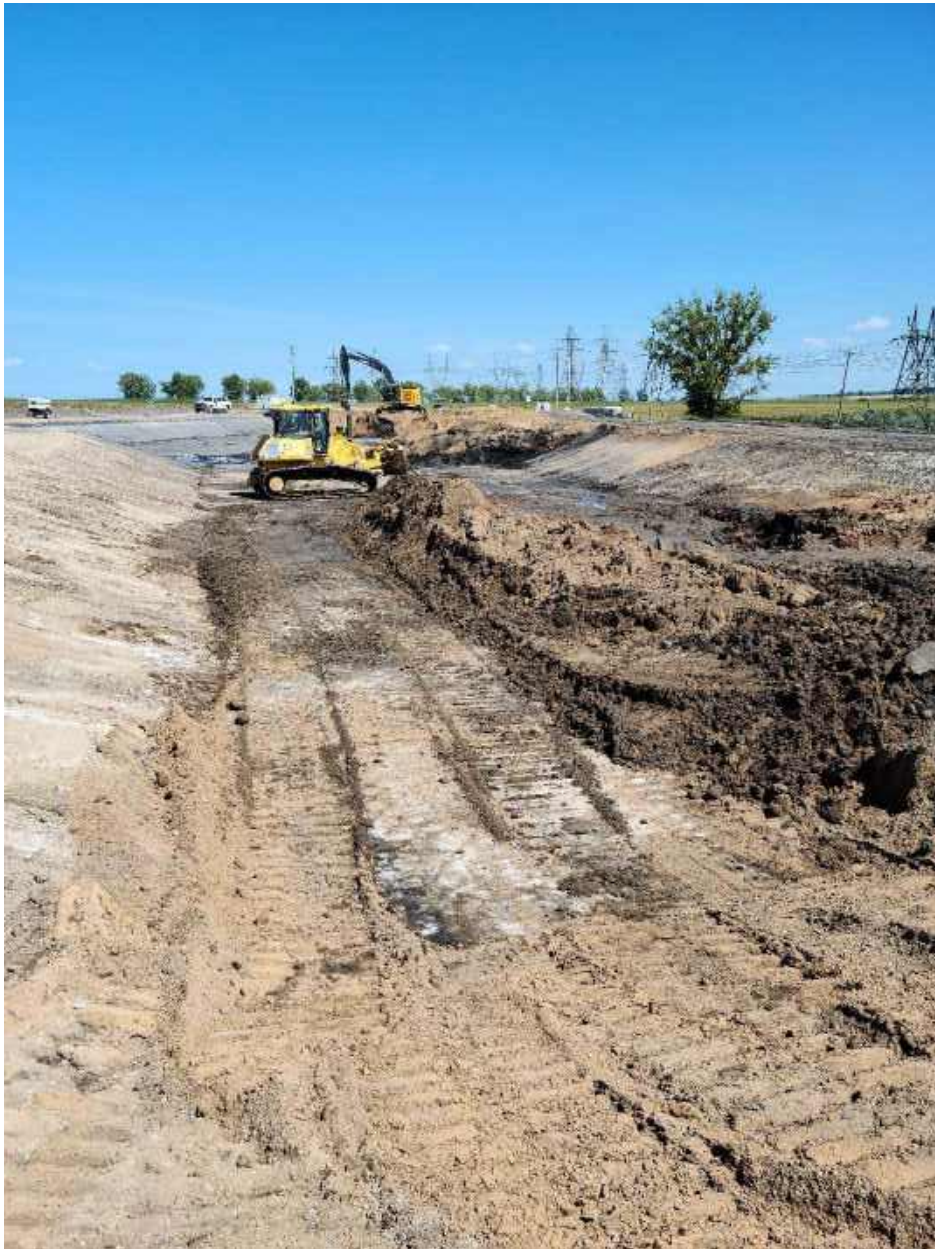
Photo 1: Fisher cleaning the ash/sand mix in the concrete-lined portion of the Settling Basin.
