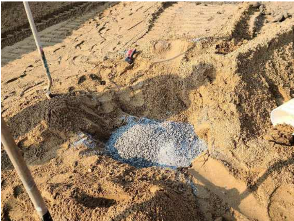
Photo 2: The remaining OW-12 casing was backfilled with granular bentonite.
