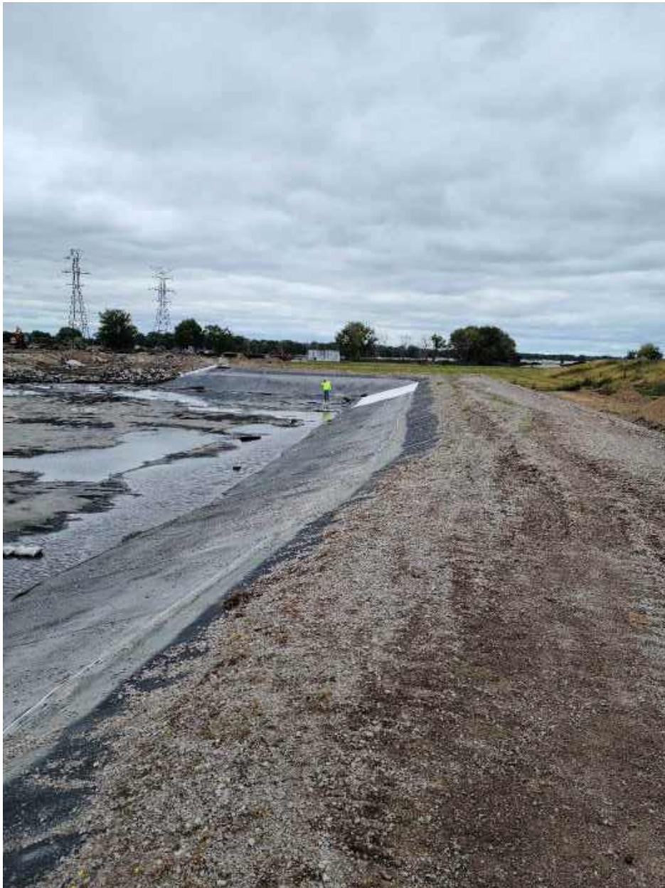
Photo 1: Fisher started removing the geomembrane liner from the Settling Basin.
