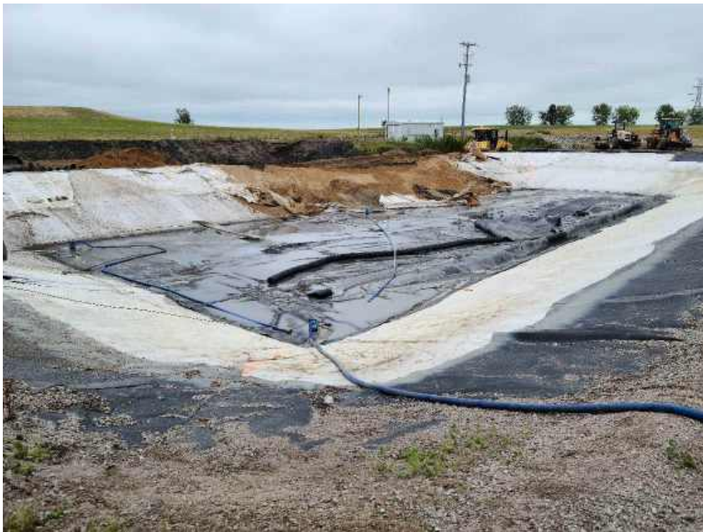
Photo 1: Fisher removing geomembrane liner and GCL from the Polishing Basin.
