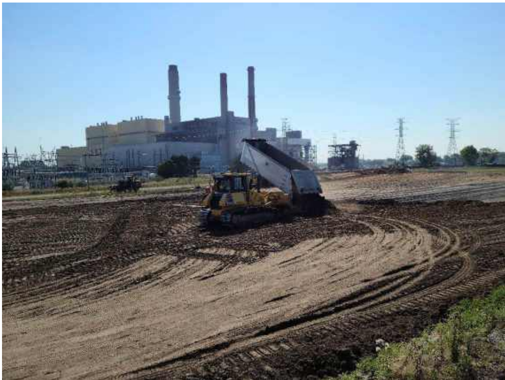
Photo 2: Fisher placing topsoil over the northern portion of the restoration.
