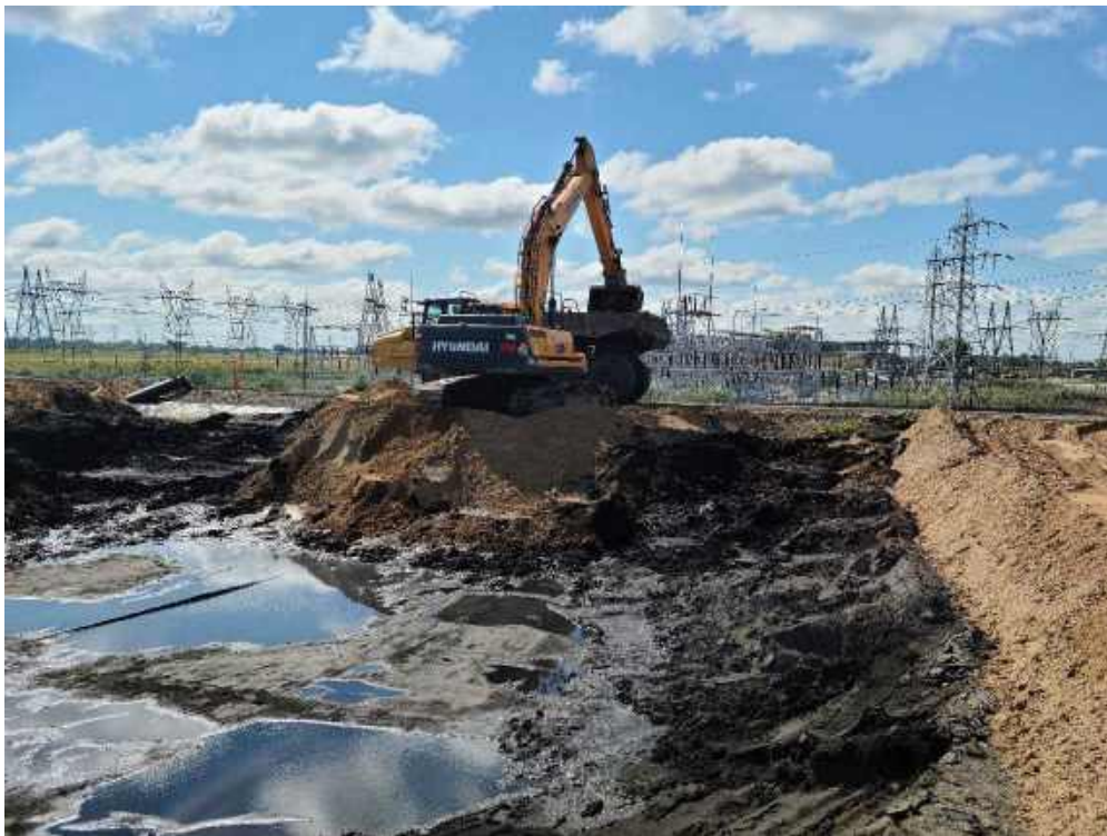
Photo 2: Fisher removing ash from the west end of the Settling Basin.
