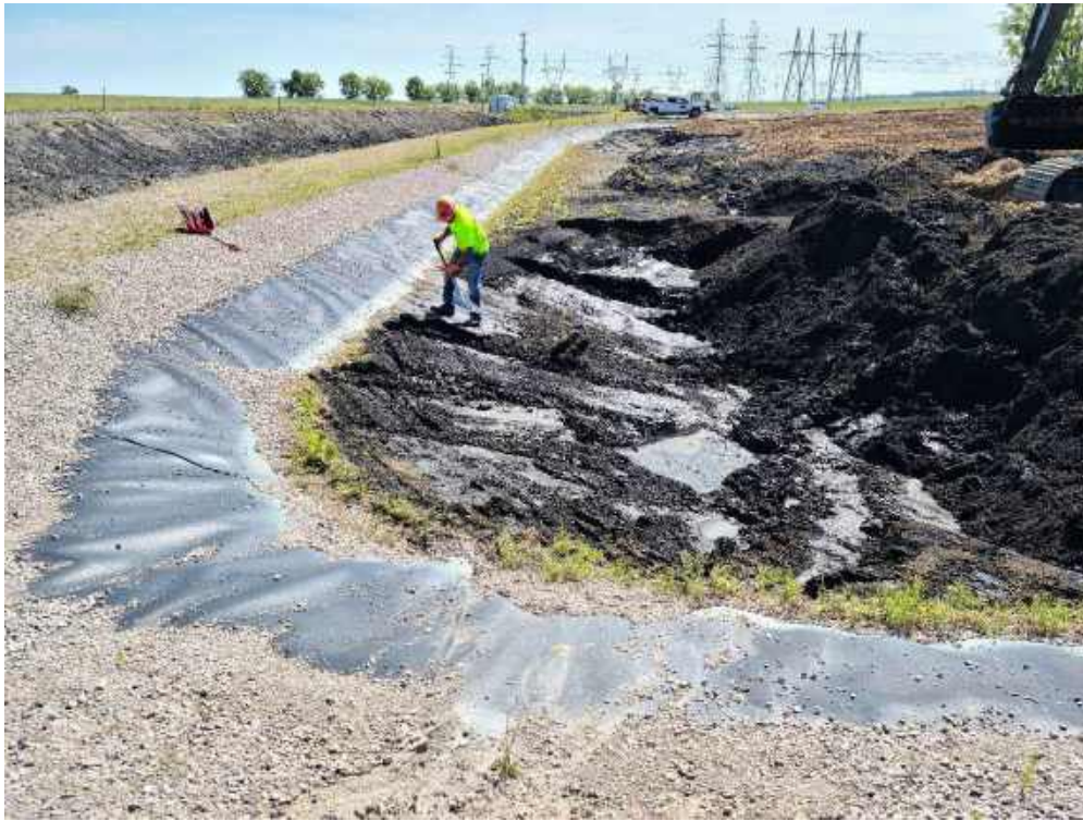
Photo 1: Fisher excavating material from the Settling Basin.
