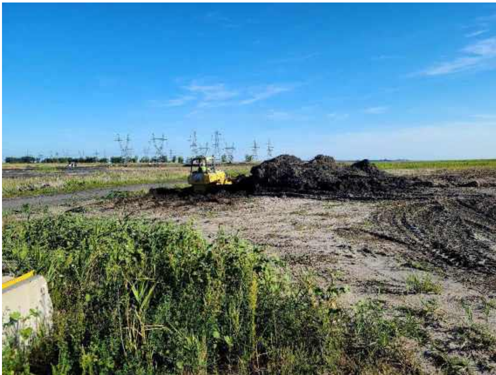
Photo 2: Fisher placing excavated material in the JCW Landfill.
