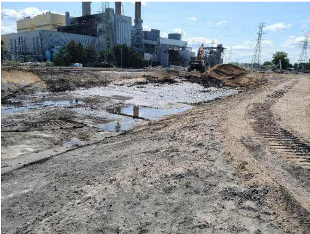
Photo 2: Fisher removing ash from the concrete-lined portion of the Settling Basin.
