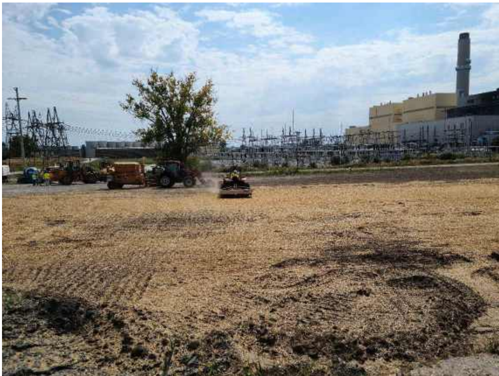
Photo 2: Fisher crimping in the straw mulch in the east end of the restoration.
