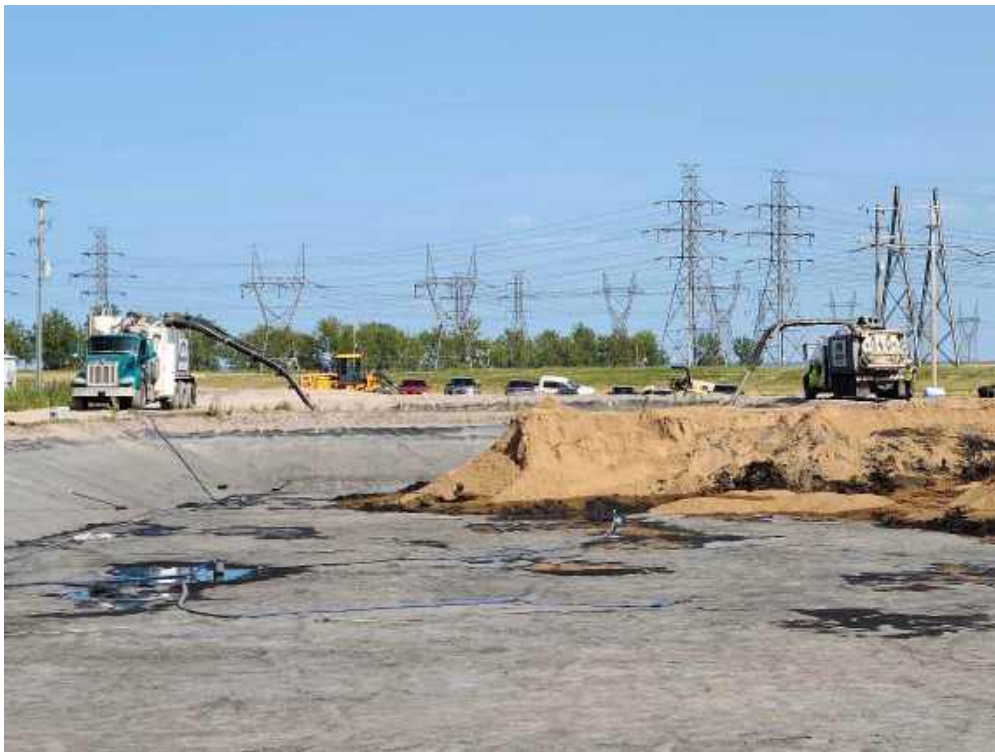
Photo 2: Fisher's progress on the Settling Basin.
