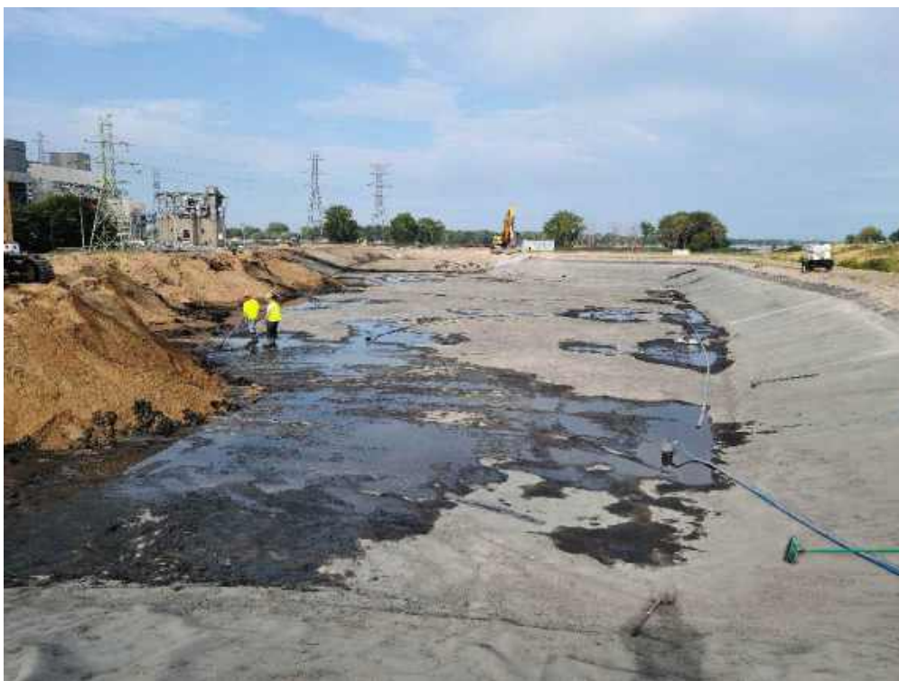
Photo 2: Fisher's progress exposing the primary geomembrane on the Settling Basin.
