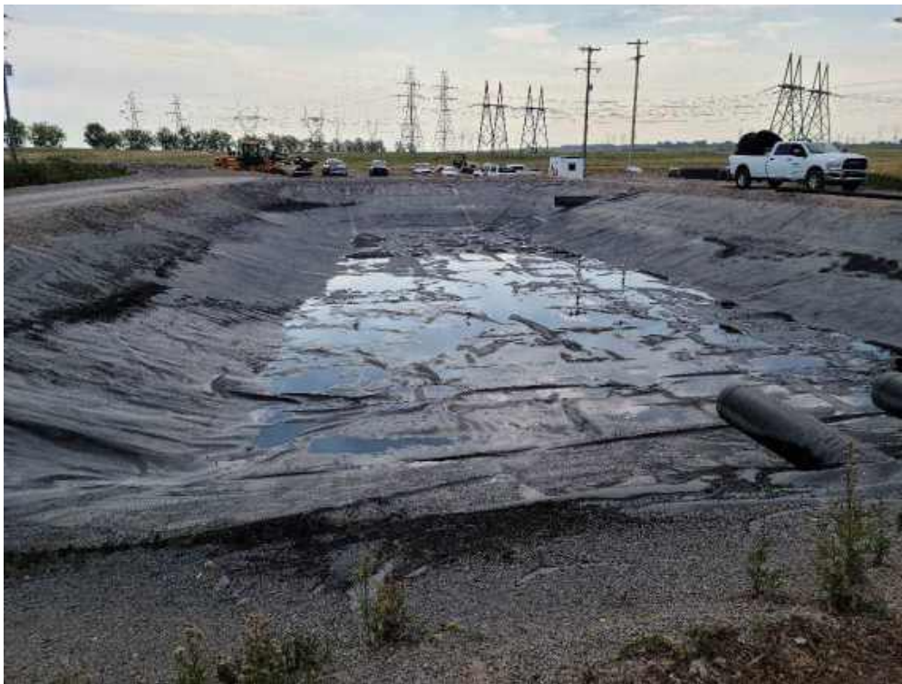
Photo 1: Polishing Basin after Badger finished cleaning and dewatering it.
