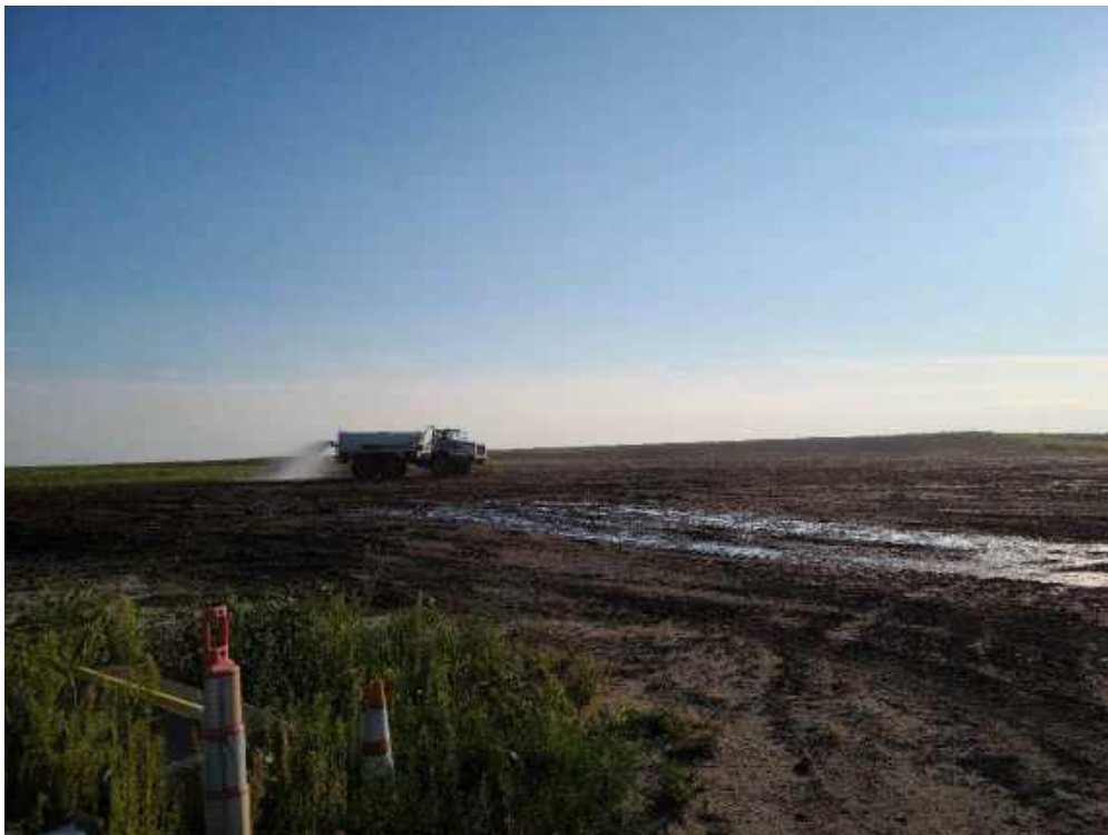
Photo 2: Fisher applying water for dust control within the J.C Weadock Landfill.
