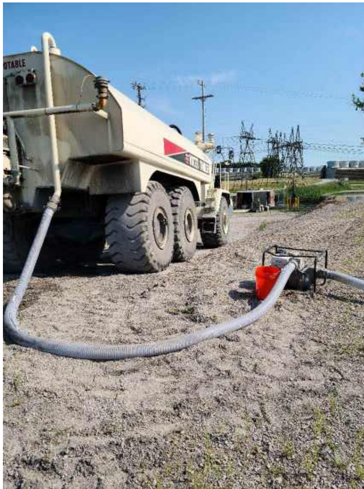
Photo 2: Fisher pumping ponded water out of the Polishing Basin.
