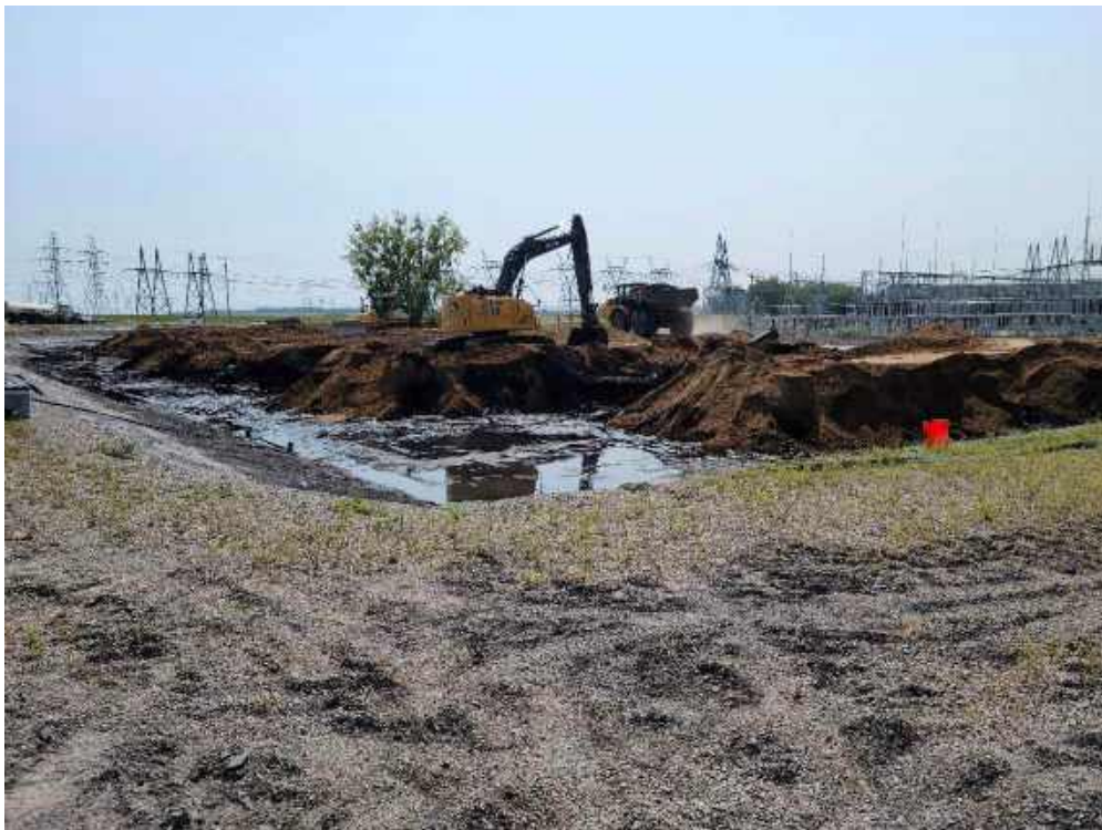
Photo 2: Progress on removal of the ash from the Settling Basin.
