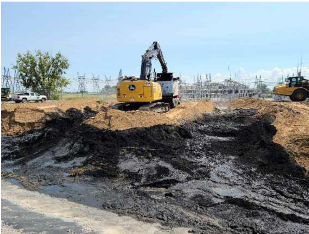
Photo 1: Fisher excavating material from the Settling Basin and loading trucks.
