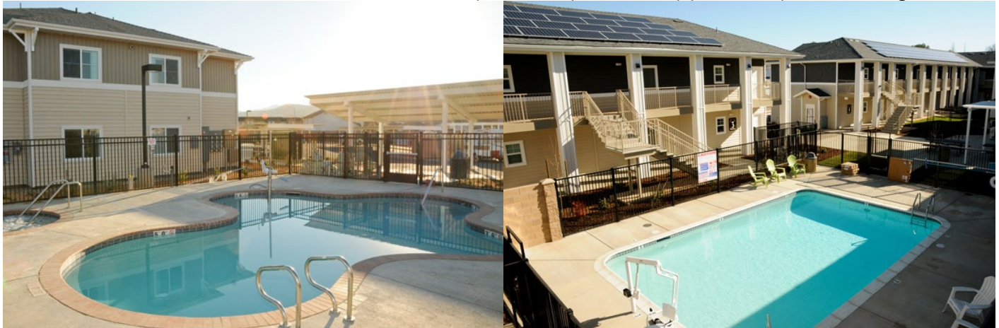
Figure 29: Pacific Companies Zero Net Energy apartment complexes built in 2014 use heat pumps for the hot tub and swimming pools (left King Station Apartments, King City, CA and right Belle Vista Senior Apartments, Lakeport, CA.)
