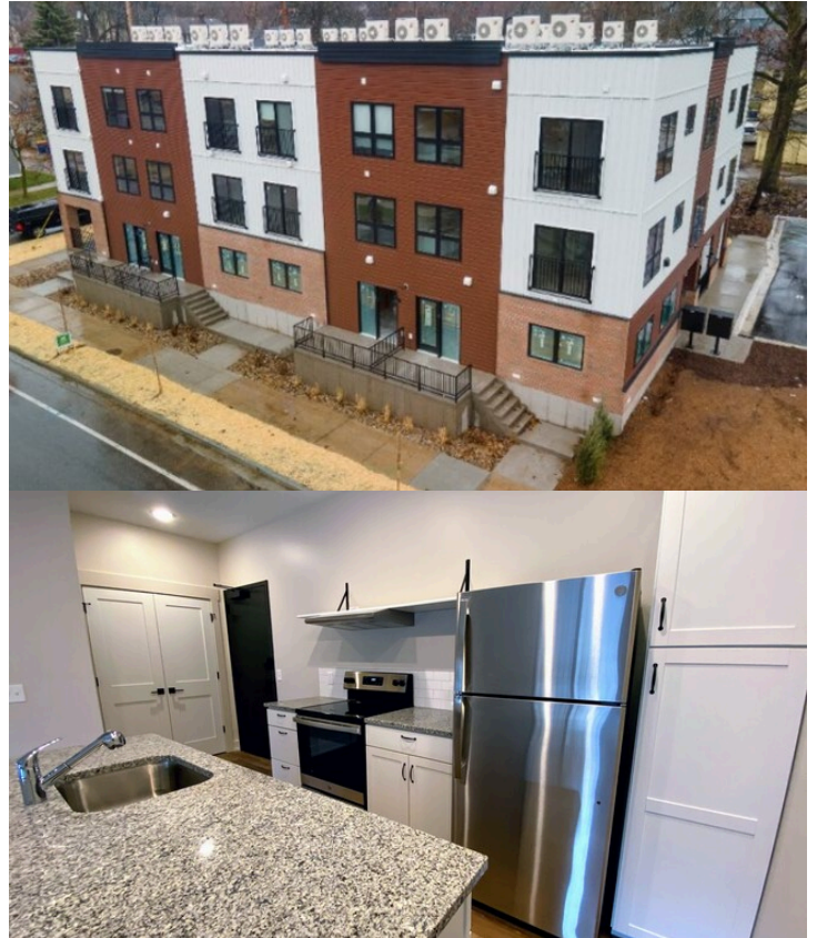
Figure 13: Bradford Station rendering and post construction in Grand Rapids, Michigan
