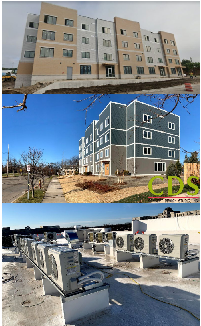
Figure 11: The Downtown Ludington Apartments in Michigan (top). The exterior view of Capital Park Apartments in Detroit and heat pumps on the roof (bottom two)
