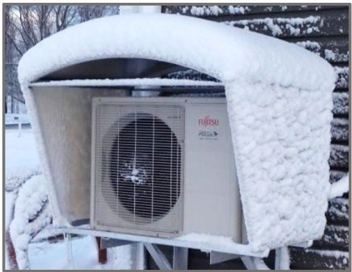
Figure 18: Air Source Heat Pumps can operate down to -31°F. 26
