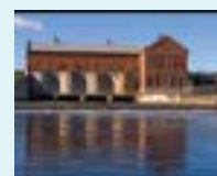
Grand River Webber Dam In-service: 1907 Capacity: 3.225 MW
