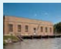
Kalamazoo River Calkins Bridge Dam In-service: 1936 Capacity: 2.55 MW
